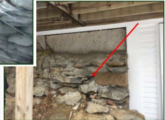
Photo #28: The stone foundation on the north side. Note the deteriorated mortar.
