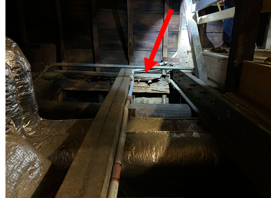
Rotted spandrel beam
