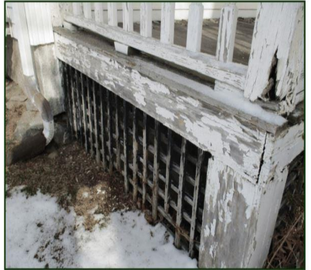
Photo #6: View of deteriorated wood at front porch
