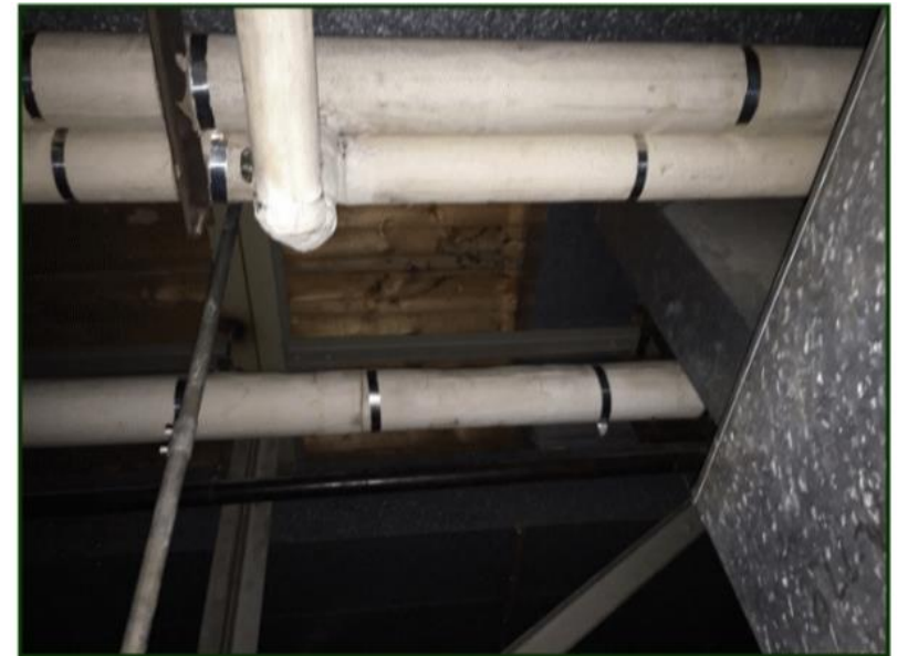
Photo #127: Photograph depicts general view of asbestos-containing pipe insulation above ceiling area in hallway
