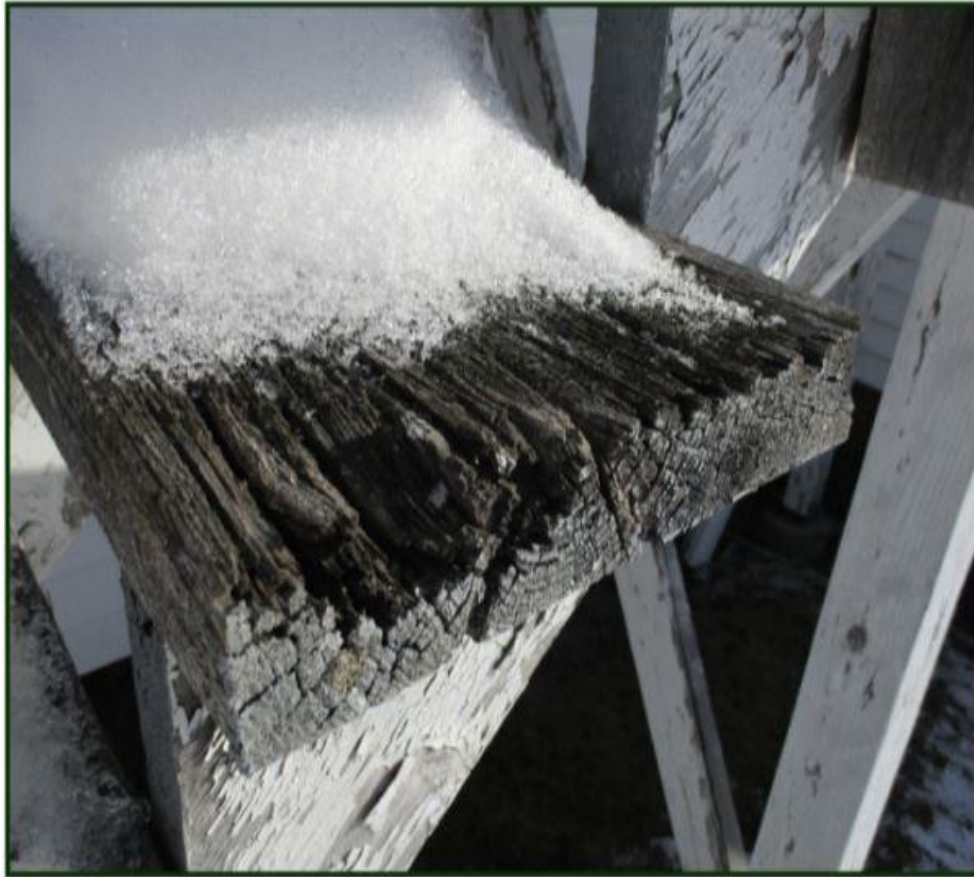
Photo #5: View of deteriorated wood at fire escape
