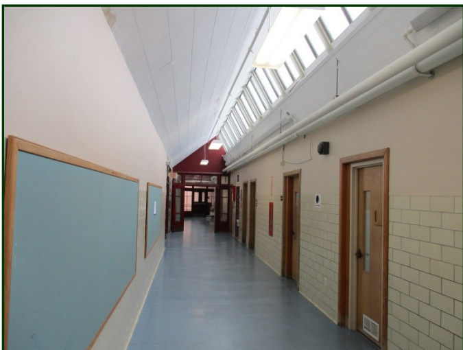
Photo #77: Typical corridor with clerestory windows, glaze faced CMU and painted plaster walls & resilient floor tile
