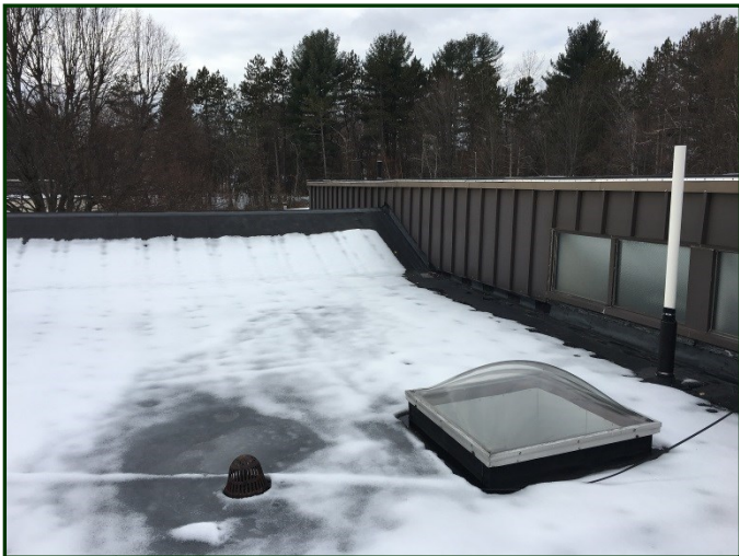
Photo #45: The EPDM roof at the north wing of the building.
