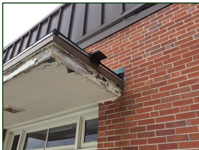
Photo #18: Detail of the entry canopy. Note the exposed wood and peeling paint.
