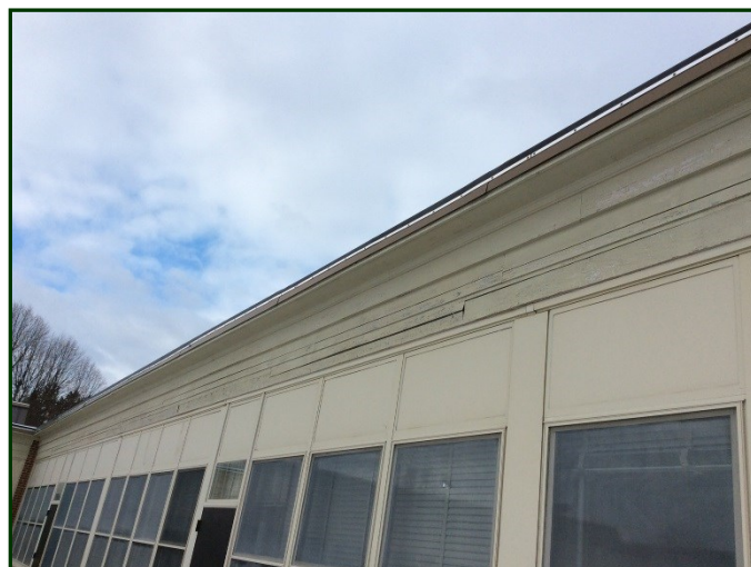
Photo #14: Wood trim over the window transoms on the north wing at the east courtyard. Note the loose board and peeling paint.
