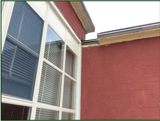
Photo #3: : Roof to wall intersection at the Cafeteria entry. Note the peeling paint at the eaves.
