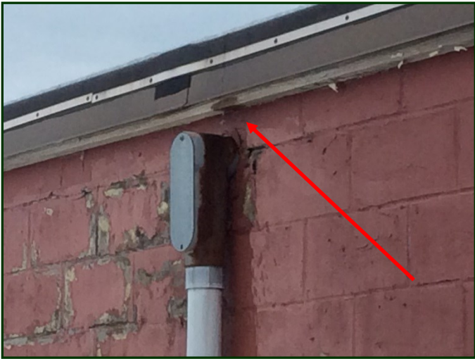
Photo #6: Detail of the emergency power conduit in the north wall. Note the water draining from the roof down the face of the wall.
