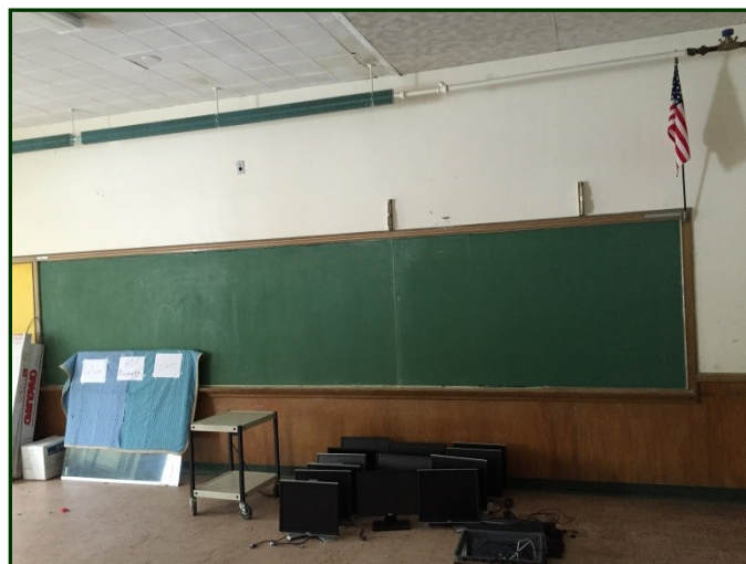
Photo #126: Photograph depicts general view of suspect asbestos-containing Chalkboards within Classroom
