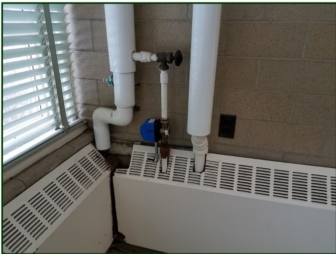
Photo #141: Typical hot water radiator and water valves in cafeteria
