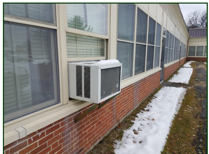
Photo #161: Typical window air conditioning unit
