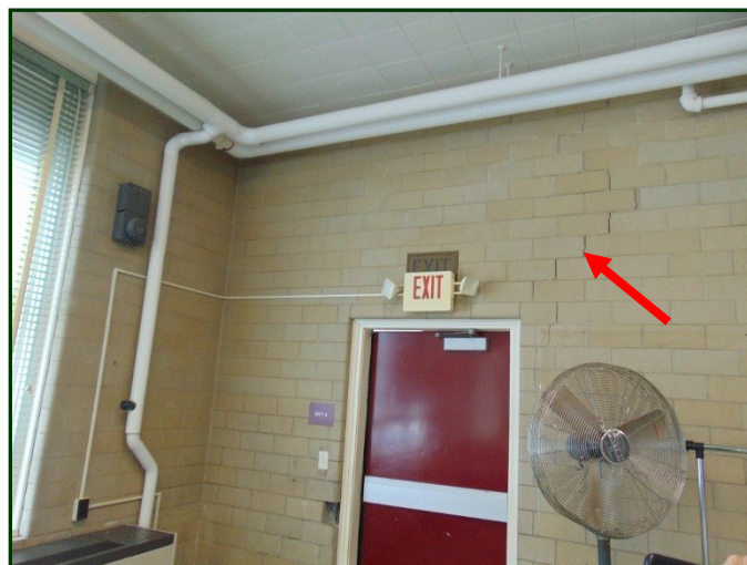
Photo #116: View of a step crack in the cafeteria.
