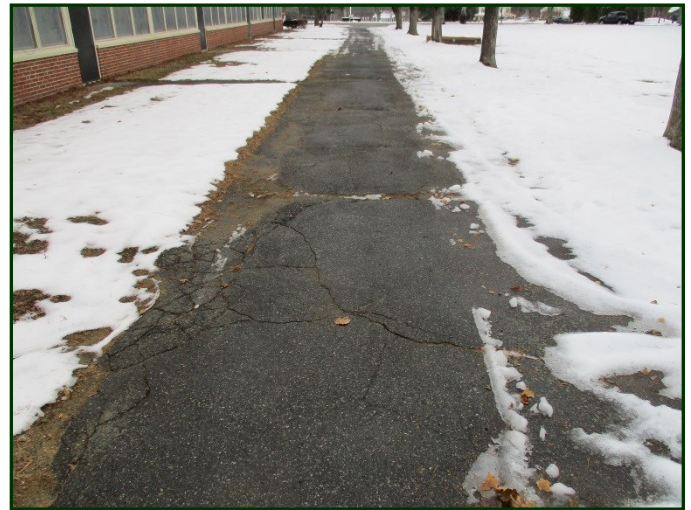
Photo #106: Deteriorated asphalt-paved sidewalk at south side of west wing
