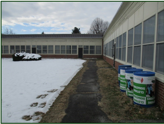
Photo #103: Deteriorated asphalt-paved sidewalk at south side of north wing
