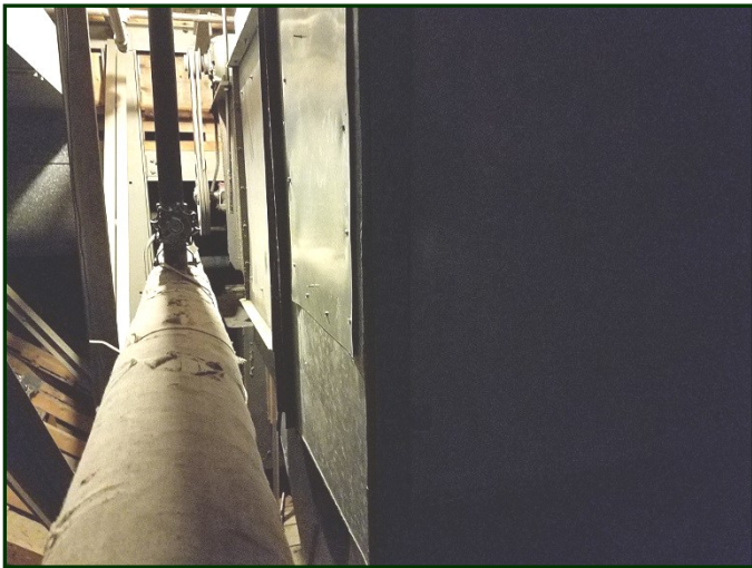
Photo #133: Typical main ventilation AHU above ceiling of corridor. Note no adequate space for routine maintenance
