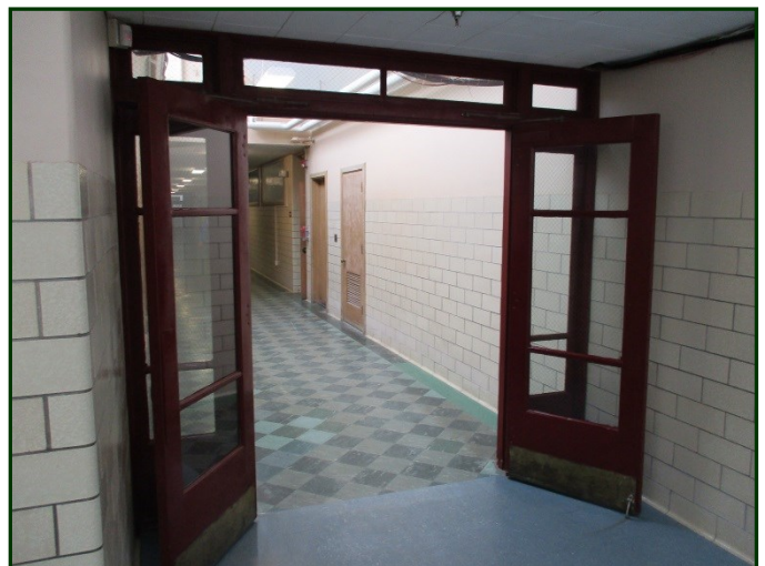
Photo #78: Corridor smoke compartment doors (south wing)
