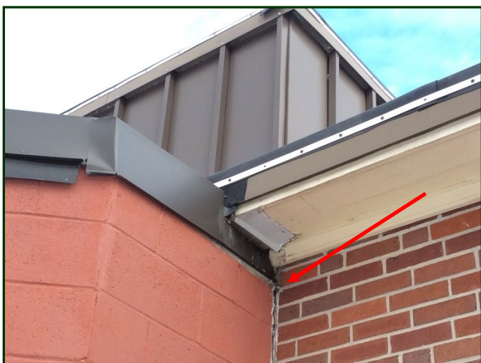
Photo #35: Intersection of CMU and brick walls at the west courtyard. Note the repairs at the soffit and the deteriorated mortar at the material transition.
