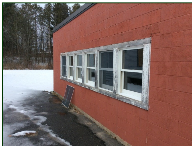
Photo #36: The west façade of the north wing. Note the peeling/missing paint at the wood window trim.
