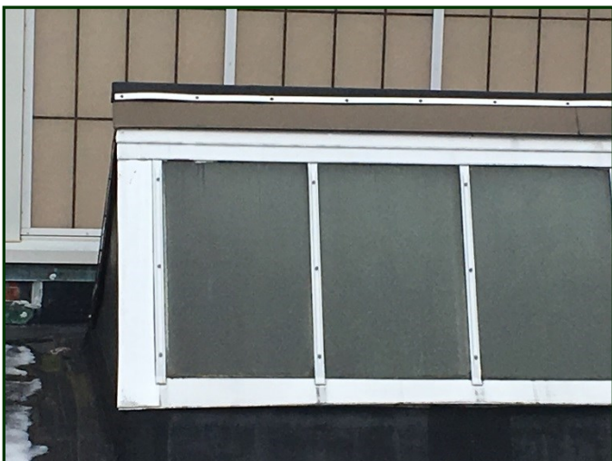
Photo #47: Detail of the main corridor clerestory windows that were clad in metal panel and topped with EPDM membrane.
