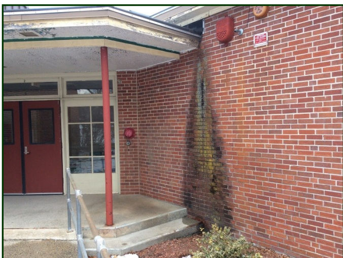
Photo #29: The secondary entrance at the southwest corner of the building. Note the staining originating from the canopy/wall intersection.
