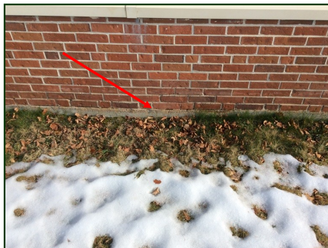
Photo #32: Detail of deteriorated mortar at the base of the wall in the west side courtyard.
