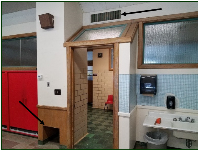
Photo #143: Typical ventilation supply register (top) and exhaust plenum (bottom) for classroom
