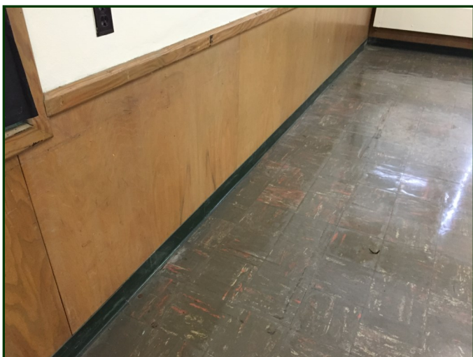
Photo #7: Photograph depicts general view of asbestos-containing 9" Floor Tile and Covebase within Classroom
