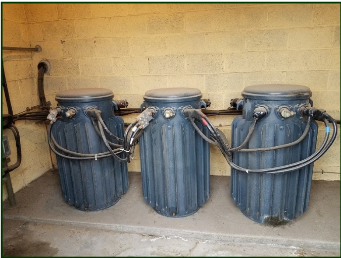
Photo #146: Main electrical transformers in electrical vault
