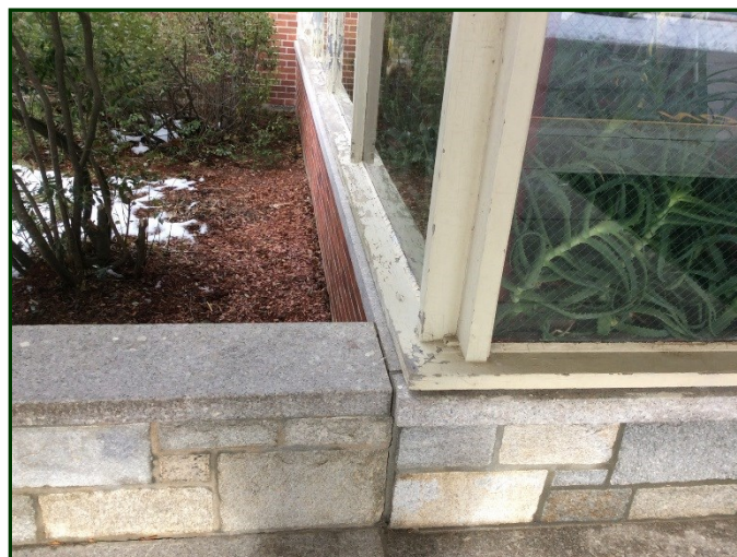
Photo #26: Detail of the wood window sill at the main entry.
