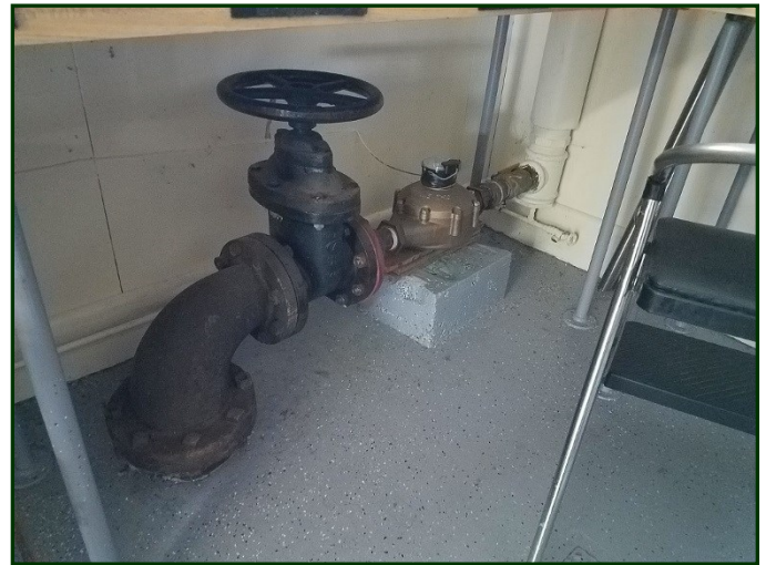
Photo #157: Main water line and meter to building
