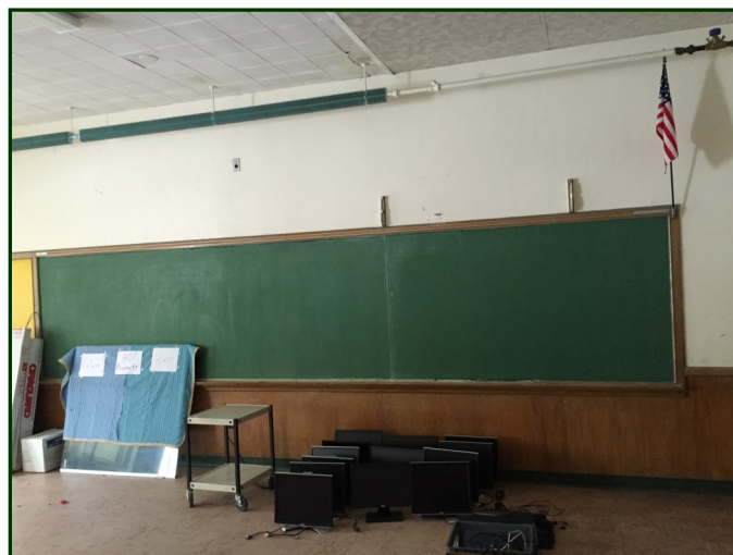
Photo #8: Photograph depicts general view of suspect asbestos-containing Chalkboards within Classroom
