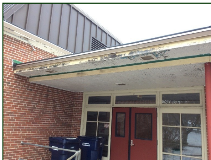
Photo #30: Detail of the canopy . Note the peeling paint and staining at the soffit and fascia.
