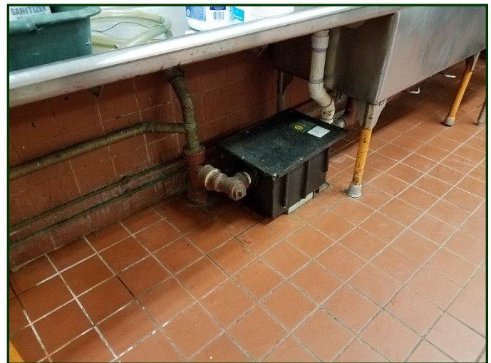
Photo #159: Grease trap at cafeteria sink
