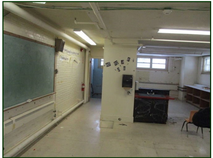
Photo #76: South side of mezzanine with painted brick walls and resilient floor tile
