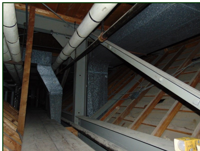
Photo #118: View of the steel truss framing supporting the roof at the northeast wing of the building.
