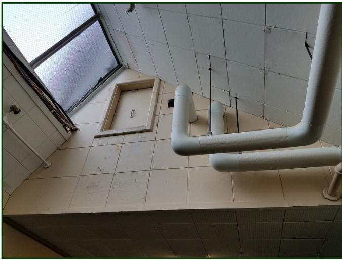
Photo #131: Access to a typical ventilation air handling unit in corridor
