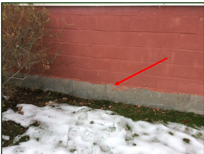
Photo #19: The east façade of the Cafeteria. Note the crack at the foundation.
