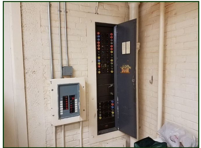
Photo #151: Square D fuse electrical panel in kitchen/breakroom area
