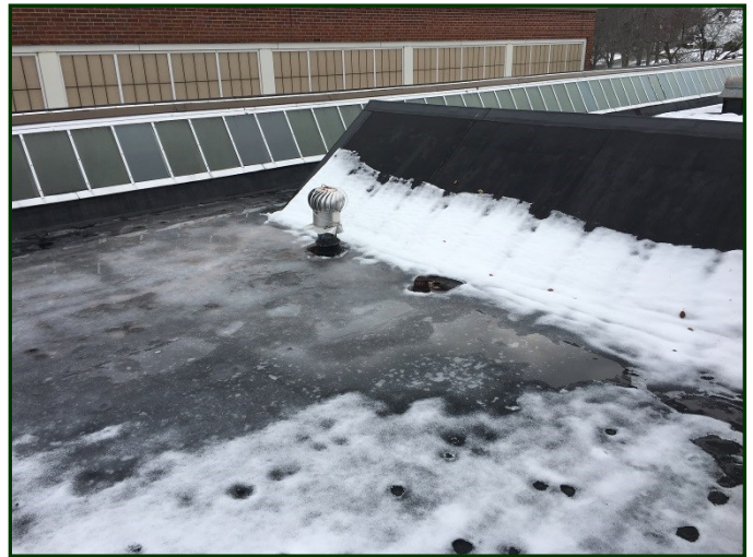
Photo #38: Roof section at the buildings central corridor showing the EPDM on the backside of the clerestory windows. Note the missing roof drain cover.
