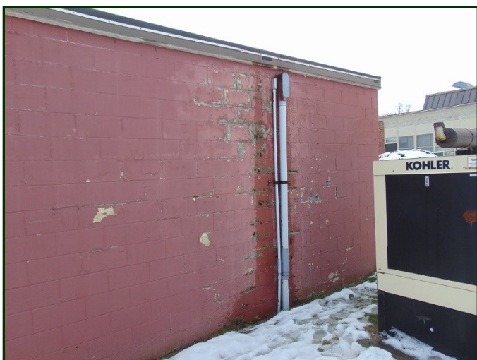
Photo #113: View of deteriorated CMU block on the north elevation of the maintenance shop.
