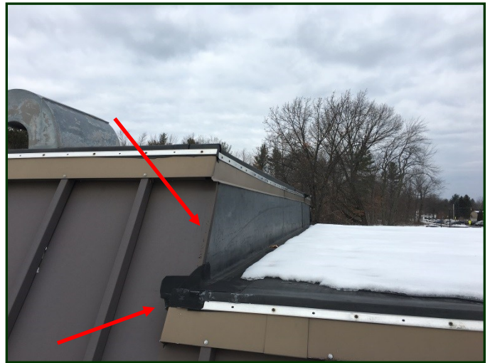
Photo #40: Detail of the standing seam panel. Note the slight rust and patch over the termination bar.
