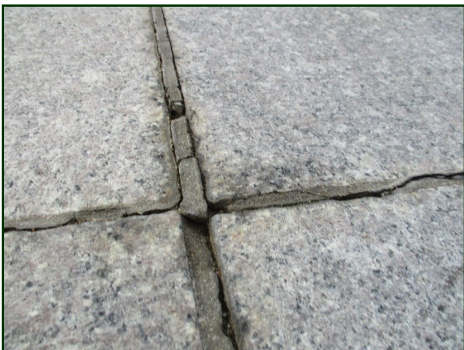
Photo #95: Close-up view of photo #94 with deteriorated mortar joints at large granite pavers
