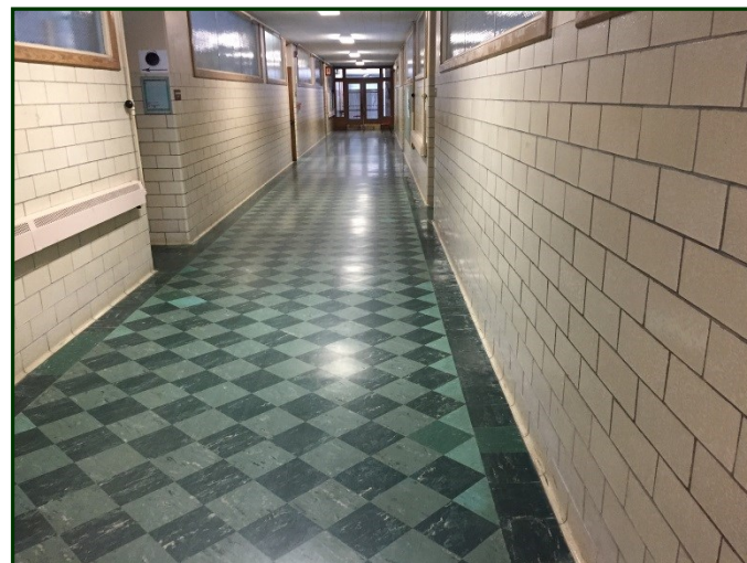
Photo #124: Photograph depicts general view of asbestos-containing 9" Floor Tile within Hallway
