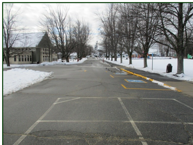
Photo #98: Asphalt-paved driveway with random cracking-south side of building (looking west)
