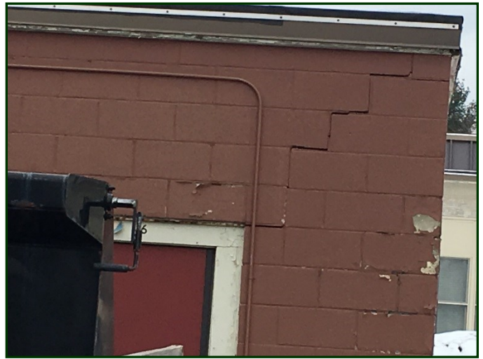
Photo #8: Detail photo of the cracked CMU at the garage.
