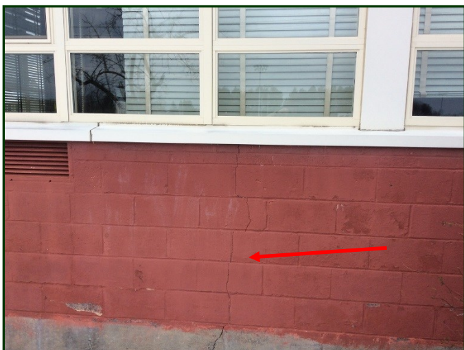
Photo #21: The east façade of the Cafeteria, Note the crack that was observed to run from foundation to top of wall.
