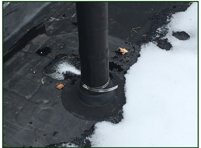
Photo #44: Detail of the pipe boot shown in photo 43.
