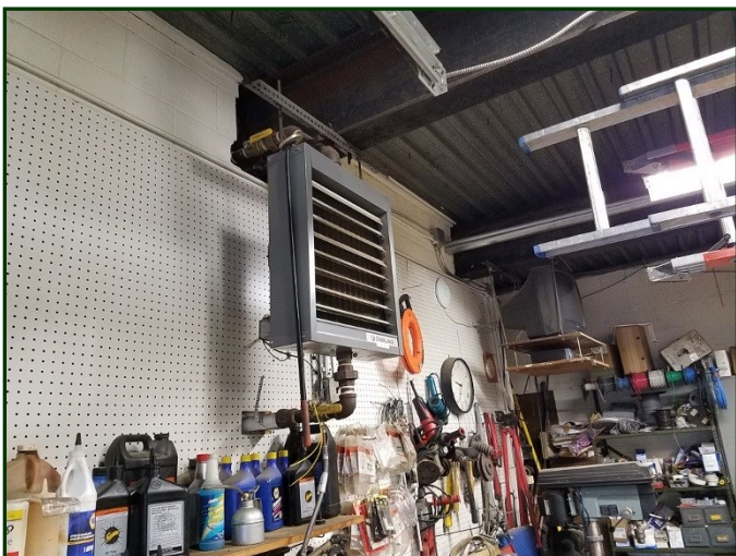
Photo #135: Typical gas-fired unit heater in maintenance shop area
