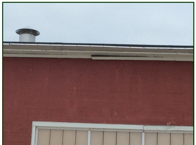
Photo #12: Loose soffit board at the Mechanical Room eave on the west façade.
