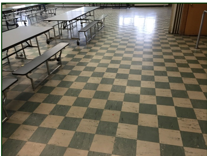
Photo #123: Photograph depicts general view of asbestos-containing 9" Floor Tile within Cafeteria
