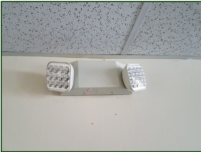
Photo #170: Backup battery lighting
