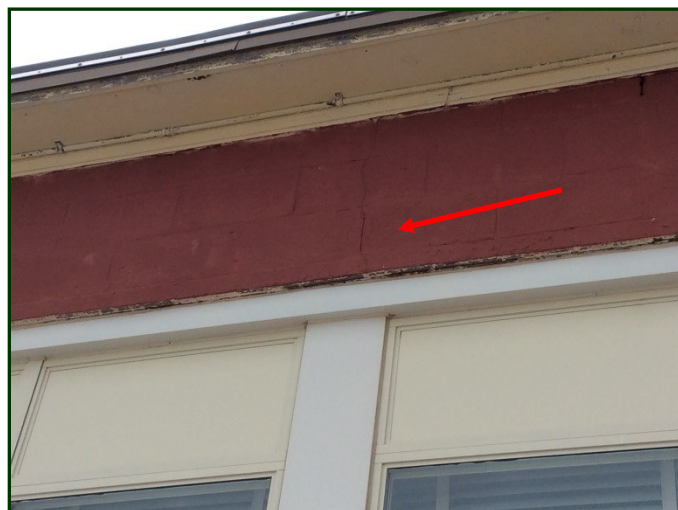
Photo #20: The east façade of the Cafeteria. Note that the crack in photo 19 continued to the top of the wall.
