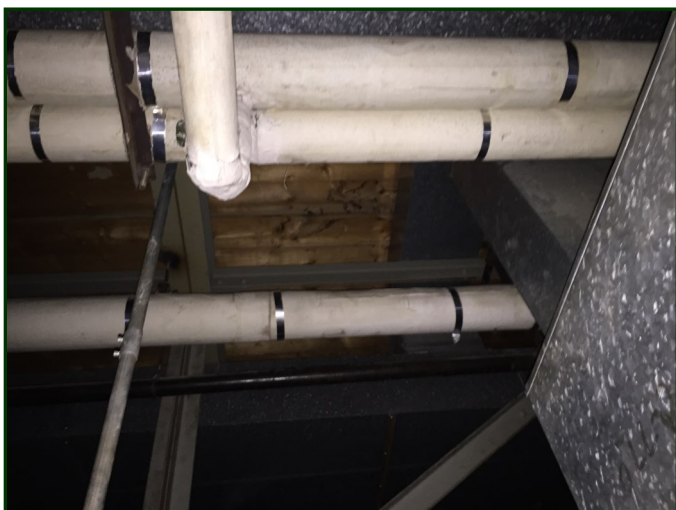
Photo #9: Photograph depicts general view of asbestos-containing pipe insulation above ceiling area in hallway
