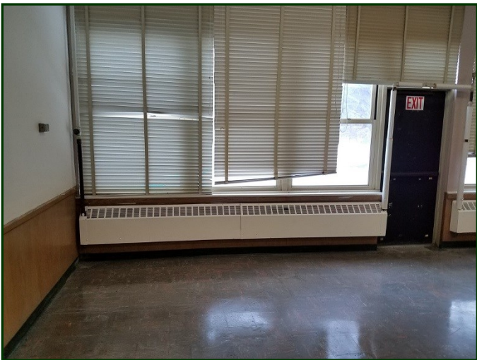
Photo #142: Typical hot water radiator in classroom
