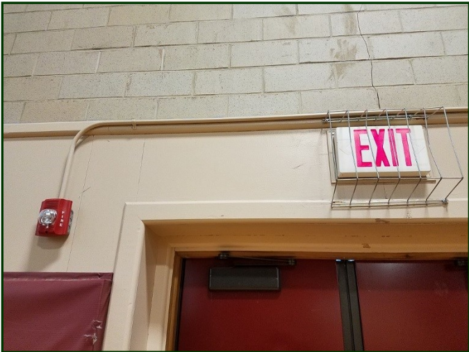
Photo #167: Typical exit sign and fire alarm strobe
