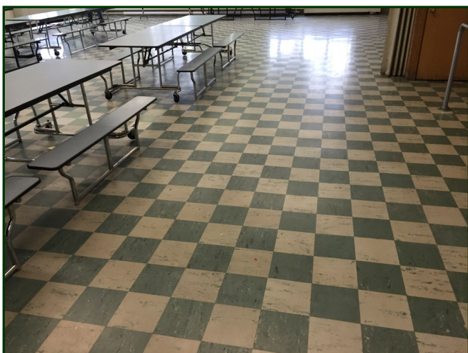
Photo #5: Photograph depicts general view of asbestos-containing 9" Floor Tile within Cafeteria
