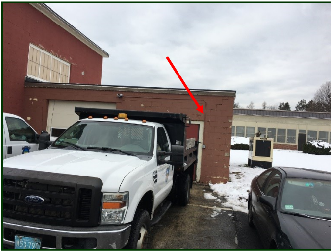
Photo #7: Maintenance garage facing east. Note the crack in the CMU wall originating from the door head.
