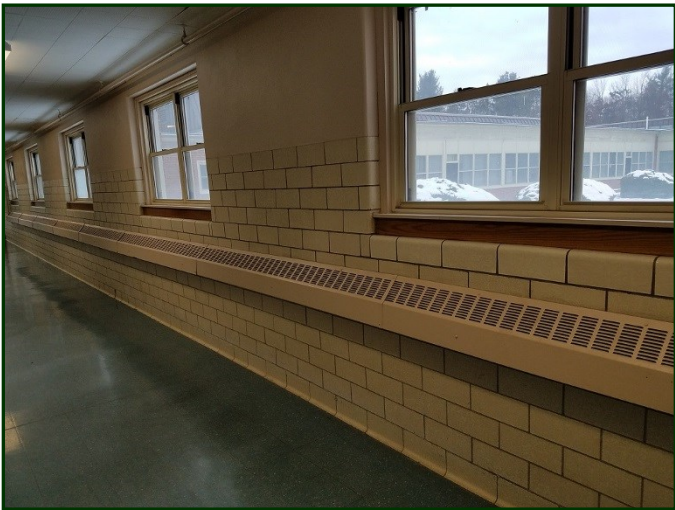
Photo #140: Typical hot water radiator in corridors
