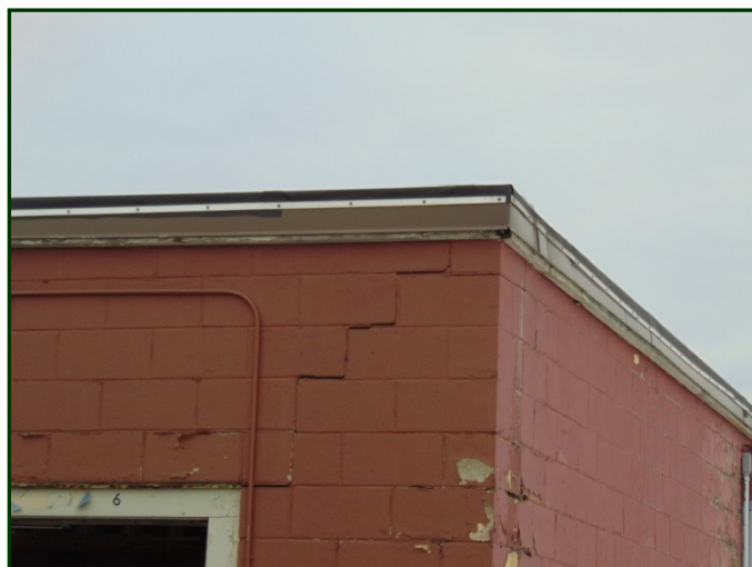
Photo #112: View of a step crack in the maintenance shop CMU wall.
