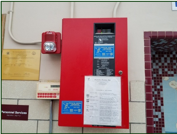
Photo #168: Fire alarm panel
