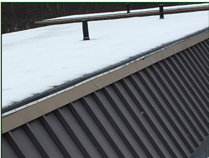
Photo #41: The top of the mechanical enclosures consisted of EPDM membrane that overlapped the edges and was secured with a termination bar at the metal panel trim.
