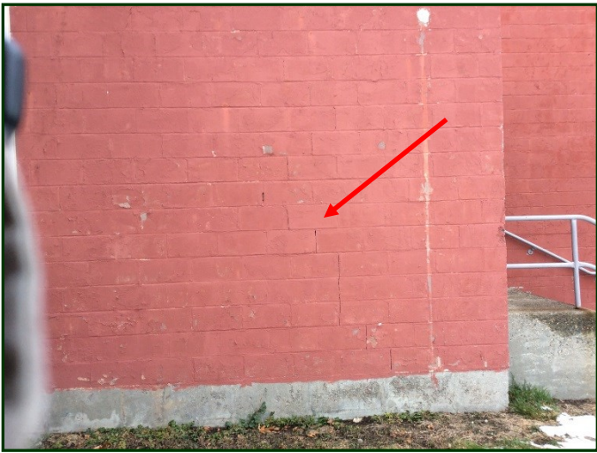
Photo #2: Crack in the south facing wall at the entry stair.
