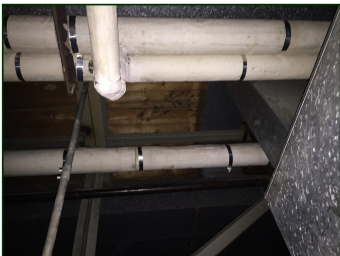
Photo #127: Photograph depicts general view of asbestos-containing pipe insulation above ceiling area in hallway
