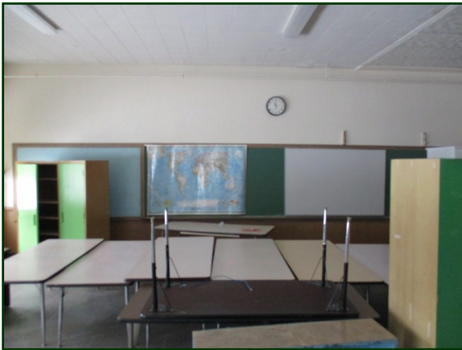
Photo #87: Classroom. Note 1' x 1' acoustical ceiling tiles (tacked on) and painted plaster walls with wood wainscot
