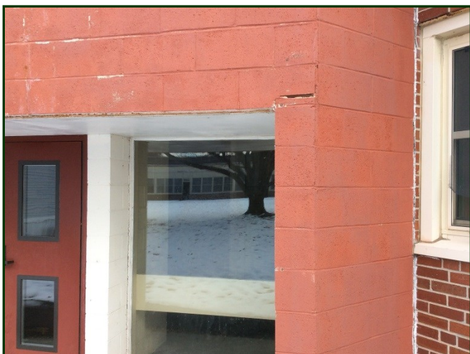
Photo #33: The building entry at the west courtyard at the north wing. Note the cracked masonry at the lintel.
