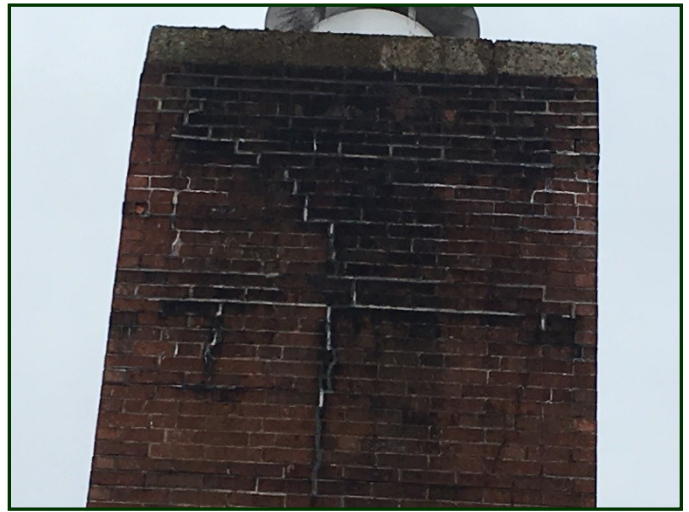
Photo #10: Chimney detail showing previous caulk repairs and some mortar cracking.
