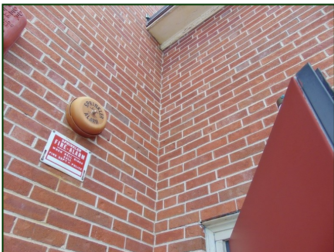
Photo #117: View of the brick exterior opposite the interior step crack. Note no visible cracks in the masonry.
