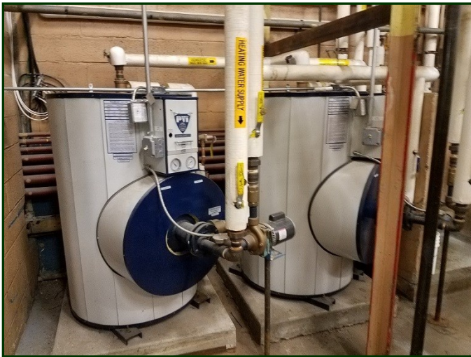
Photo #158: Domestic hot water heaters
