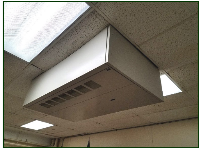
Photo #134: Ventilation AHU for kitchen breakroom area adjacent to Gym
