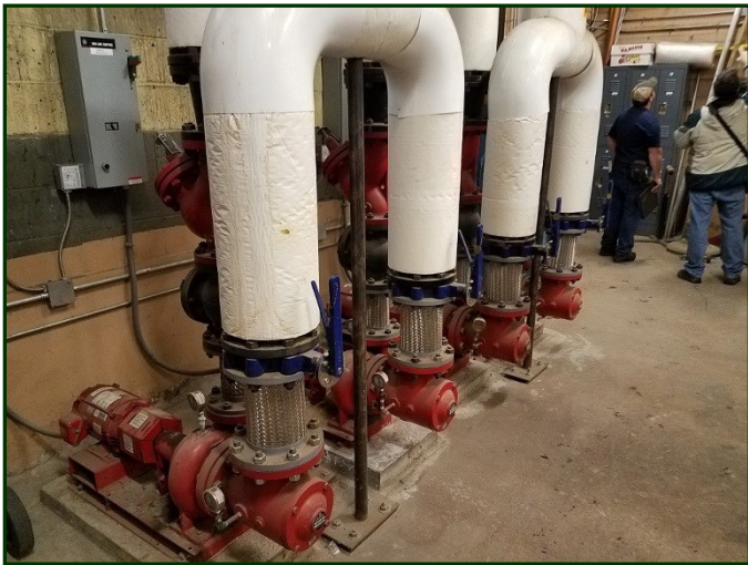
Photo #139: Heating hot water pumps
