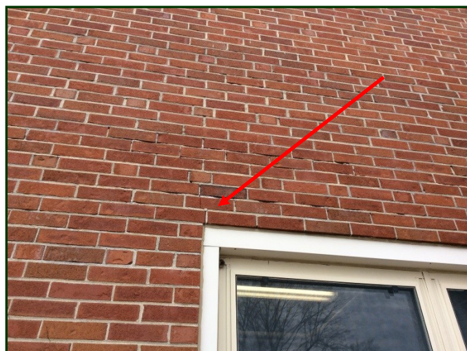
Photo #24: Detail of the window head of the window in photo 23. Note the cracked brick and the deteriorating mortar.
