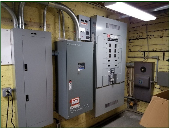
Photo #148: Secondary electrical panels and automatic transfer switch for generator
