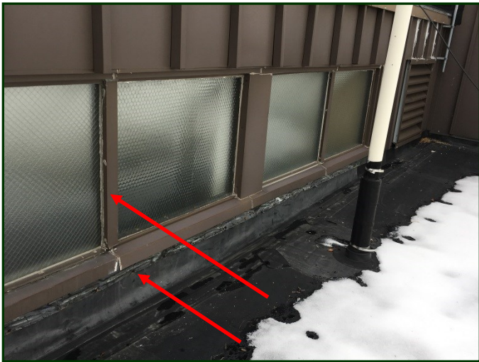
Photo #43: The clerestory windows at the north wing. Note the brittle sealant and rusted fasteners at the counterflashing.
