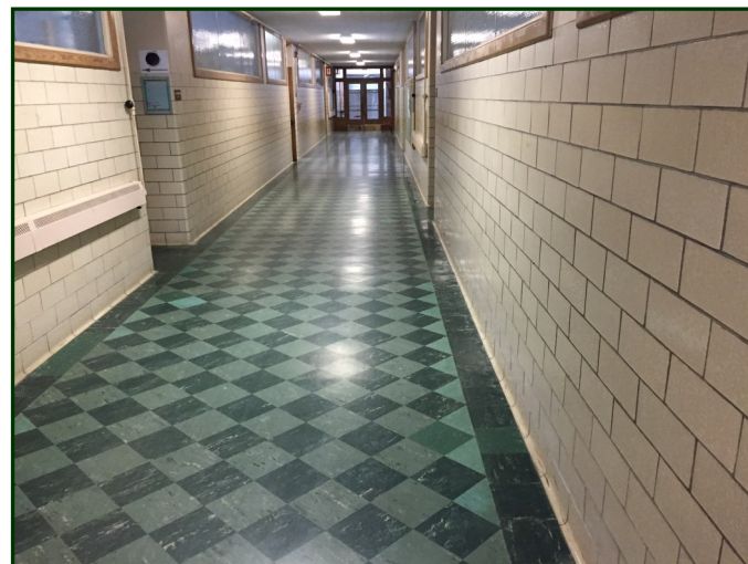
Photo #6: Photograph depicts general view of asbestos-containing 9" Floor Tile within Hallway
