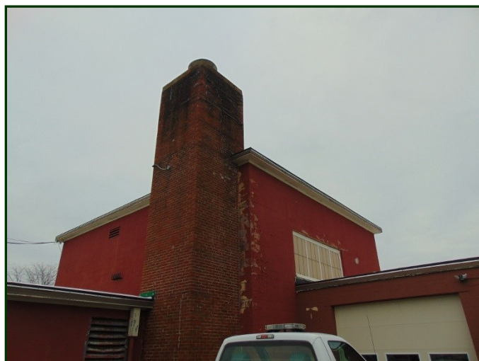
Photo #110: View of the brick chimney on the east side of the building. Note staining around chimney.
