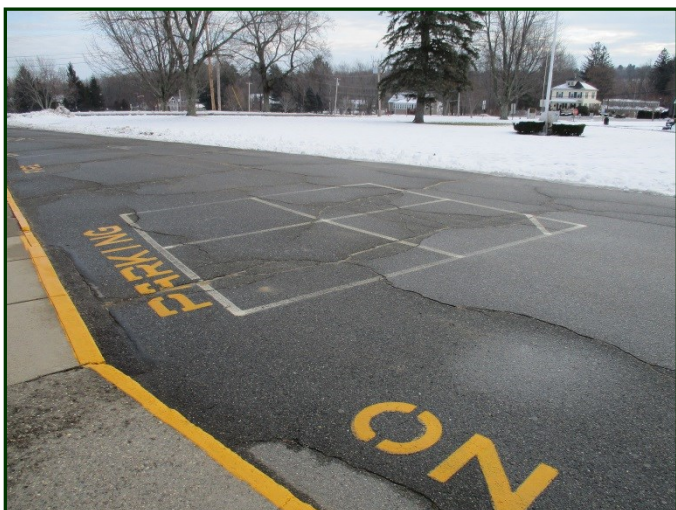
Photo #97: Asphalt-paved driveway with random cracking-south side of building (looking east)
