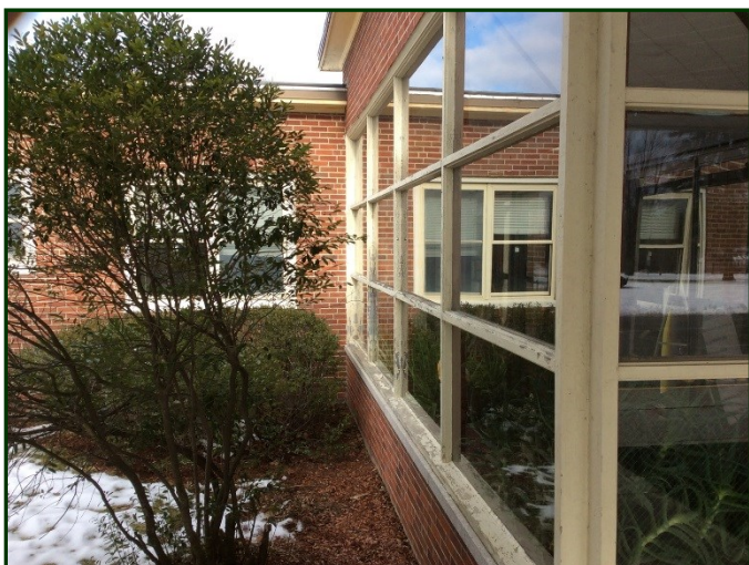
Photo #27: Wood framed glass vestibule. Note the peeling paint.
