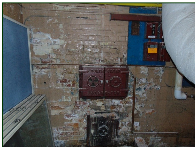
Photo #114: View of the brick chimney from the interior. Note the peeling paint and deteriorated mortar joints.
