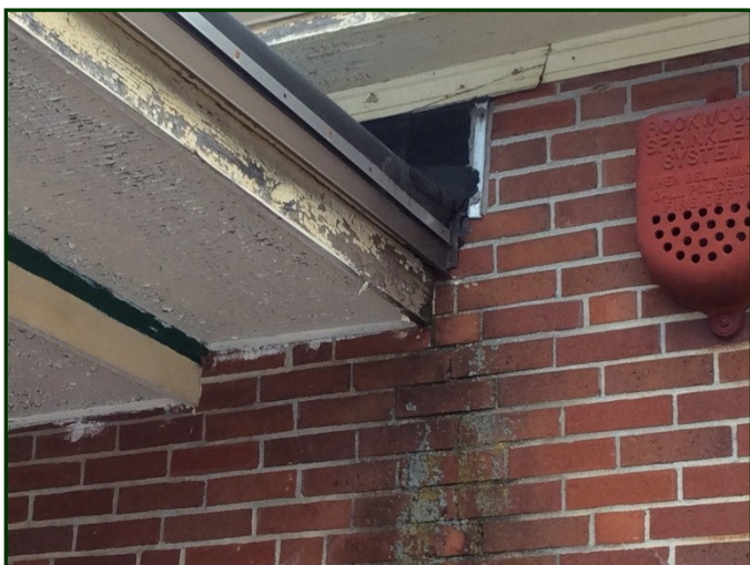
Photo #31: Detail of the canopy intersection at the brick wall. Note the deteriorating mortar under the soffit.
