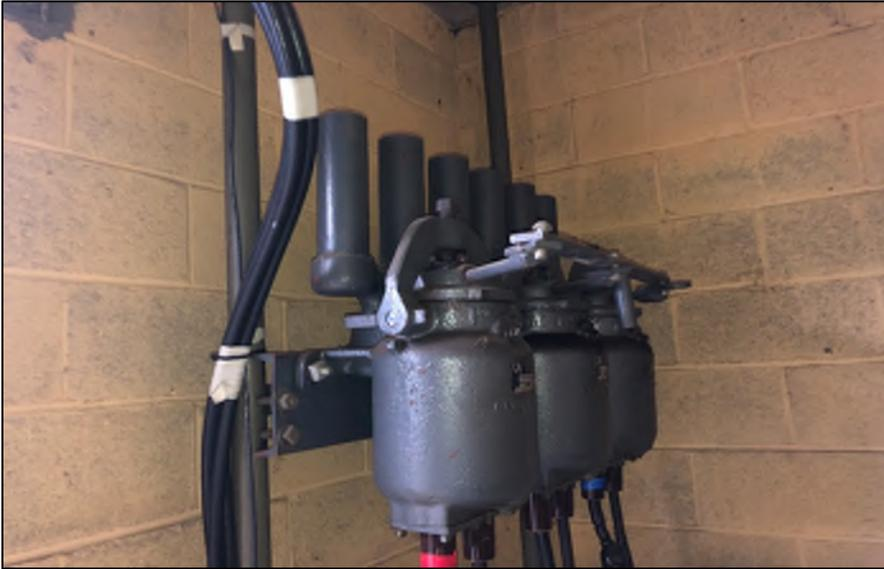
Photo 9: Old oil-filled switchgear equipment associated with Passios School in the Electrical Room.
