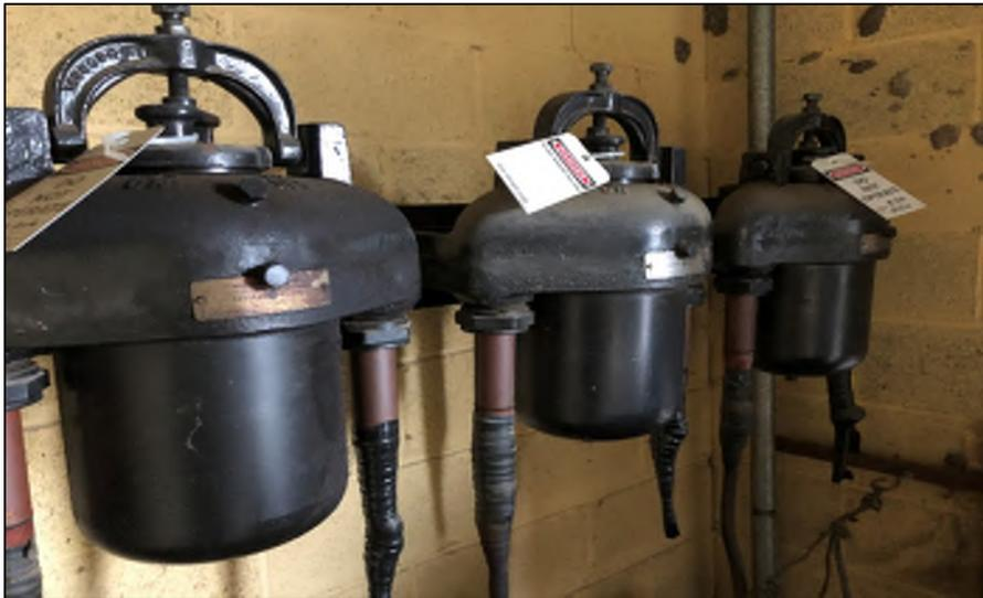
Photo 7: Old oil-filled switchgear equipment associated with the High School.
