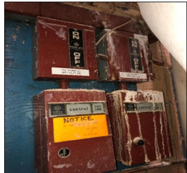
Photo 16: Old oil pump switches near the incinerators in the Boiler Room.
