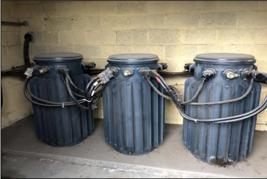
Photo 5: Blue transformers in the Electrical/Transformer Room.
