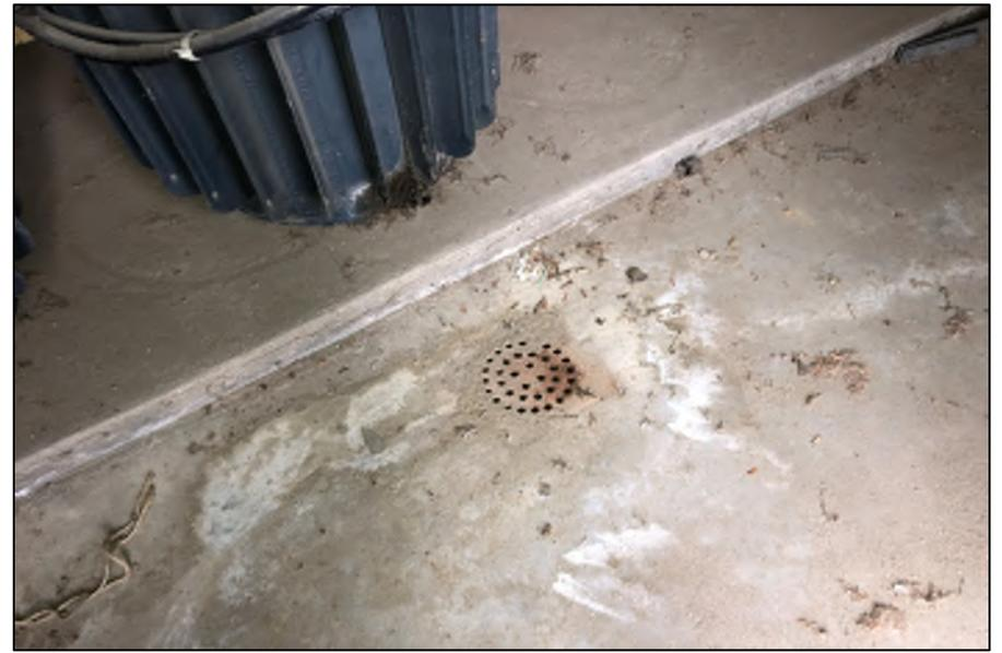
Photo 6: Floor drain adjacent to the blue transformers in the Electrical Room.
