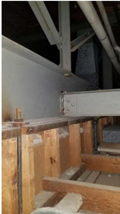
**Photo 2** Wood framed ceiling hung from structural steel above corridor.
