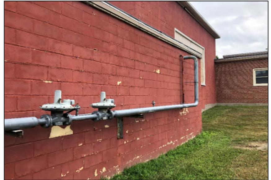
Photo 28: Natural gas piping on the side of the Maintenance Garage.
